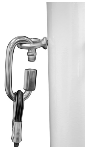
Figure 19. Attaching the guy wire carabiner to the tower structure eye screw
